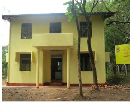
New Vidatha Building
