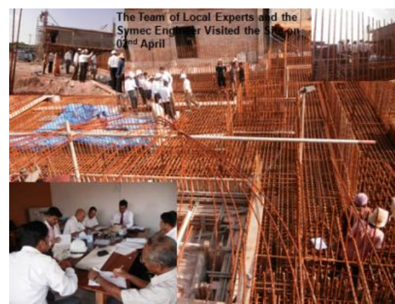
Supervision of installation of all the EPs
