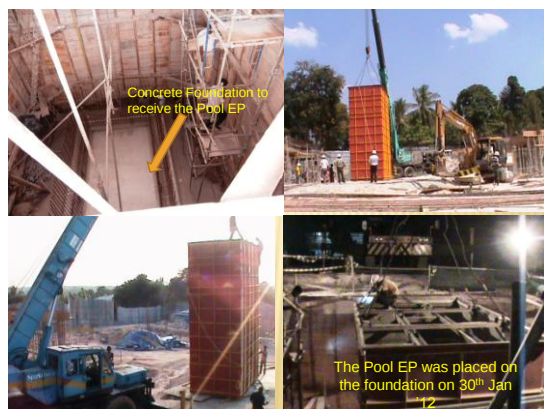
The concrete foundation prepared to receive the Pool EP.
