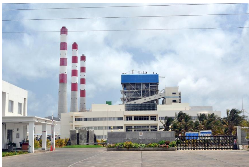
Fig 9 – Puttalam Coal Power Plant
