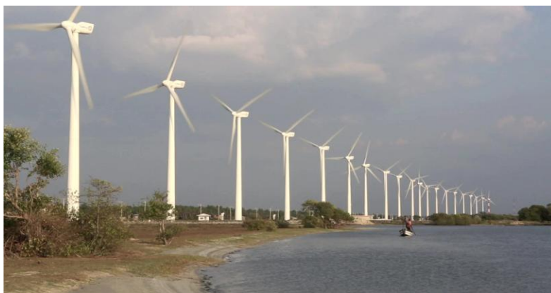
Fig – 11 –Wind Power Plant - Puttlam
