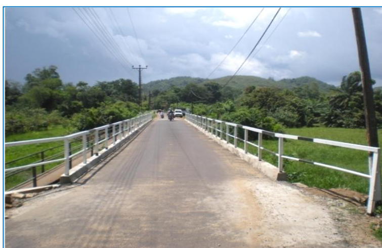
Repaired Bridge at Thebuwana - Kalutara
