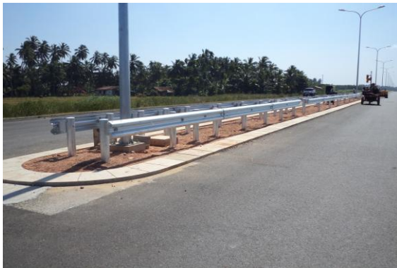
Fixing of Guard Barrier fence
