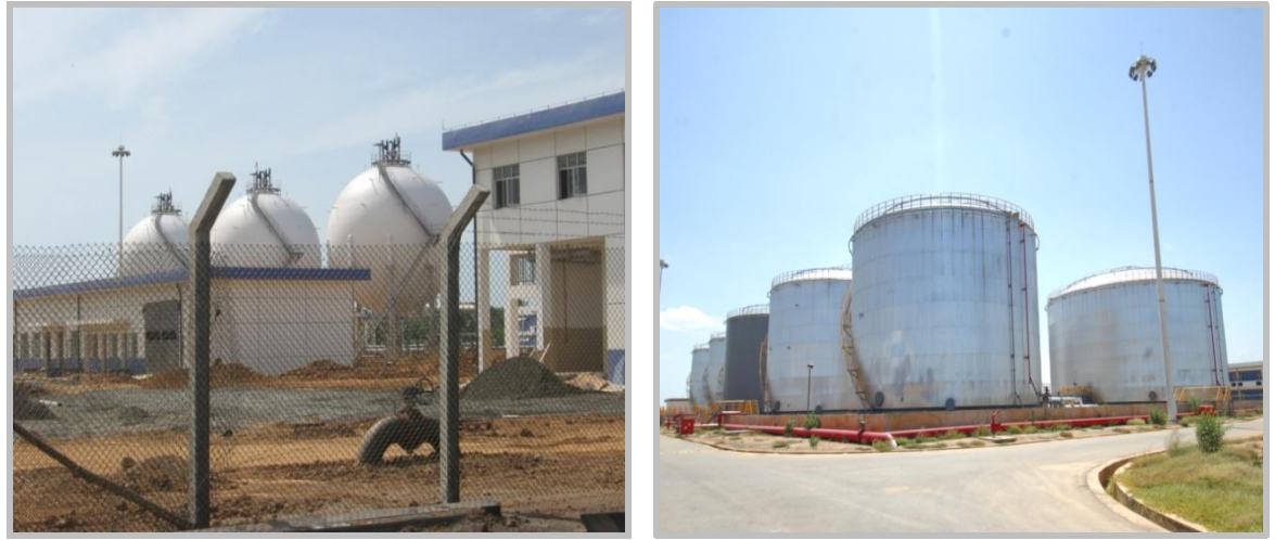
Bunkering Facilities and Tank Farm Project in Hambantota
