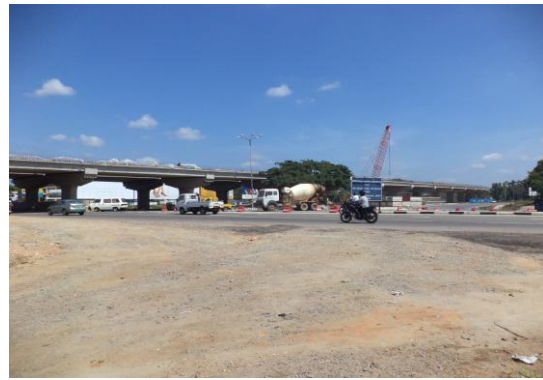
Construction of Katunayaka Via duct
