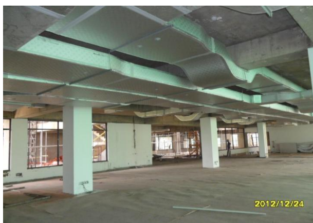
Air Condition ducting works in progress
