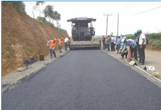
Construction works of Hatton – Nuwara-Eliya Road
