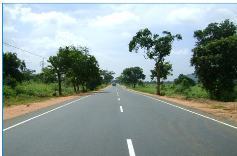
Kanthale – Trincomalee Road Section
