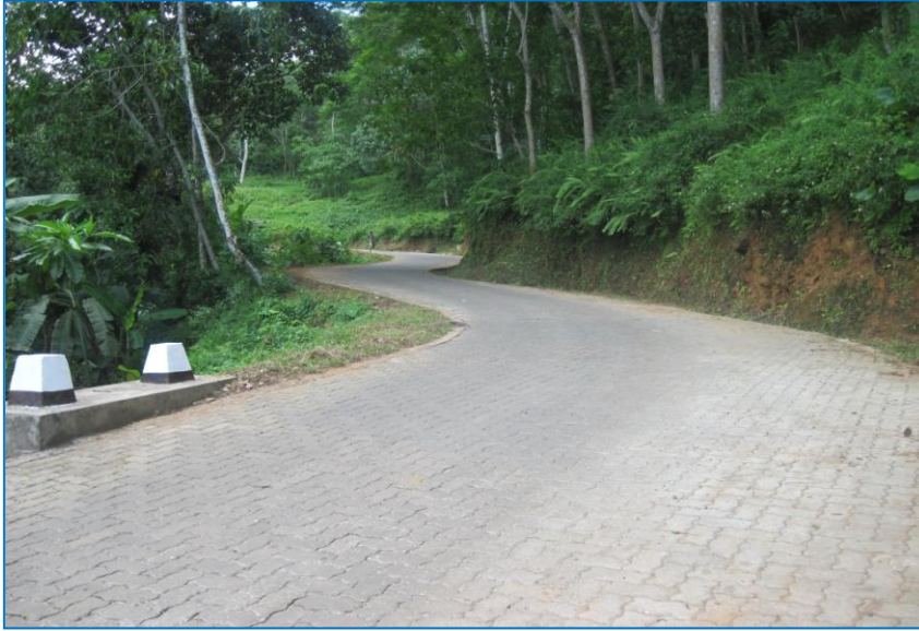
Magala to Deraniyagala road - Kegalle
