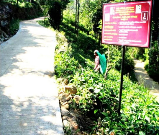
Recently completed 'Nadsa road No. 09, under MC SPMU's Intervention for Community Infrastructure Development at Parapaha in Doluwa DS Division, Kandy District.
