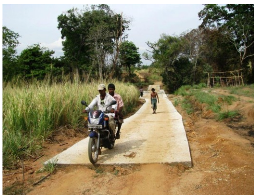
An access road assisted by SPEnDP – Monaragala under community development component (2012) at Thelabogalla, Veheragalain Moneragala District.
