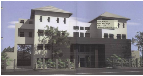
1) Courts Complex at Homagama (Proposed Building)
