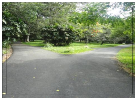
Carpeting of internal roads system
