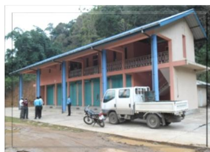
Construction of Maspenna Bus Stand in Welimada DS Division Badulla District
