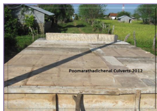
Construction of Bridge and Culvert Verugal, Trincomalee
