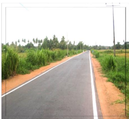
Makandura-Udawela Road, Katugampola DS Division Kurunegala District Carpeted distance - 11.38 Km
