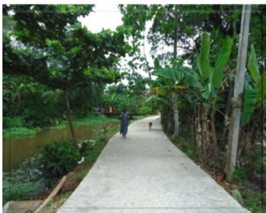
Road constructed parallel to Moragoda Canal, Maligaspe Kadawath Sathara Divisional Secretary Division Galle District
