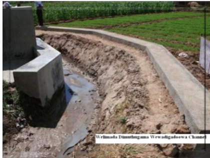
Reconstruction of Dimuthugama Wewadigodaduwa Irrigation canal Welimada DS Division
