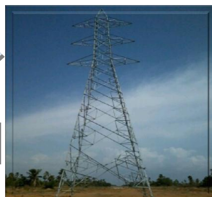
Construction of Chunnakam electricity sub station
