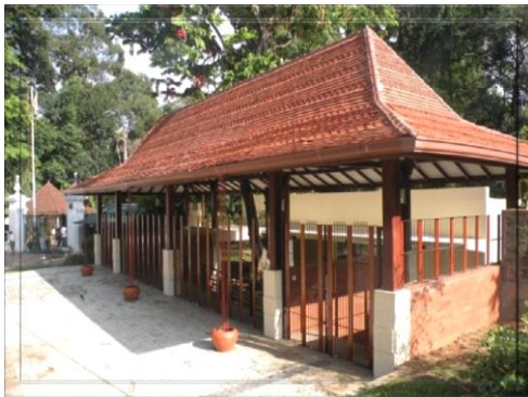
Construction of ticket counter
