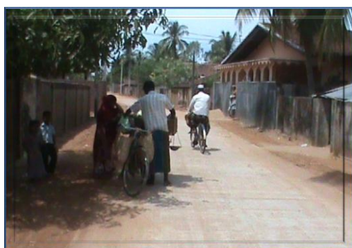
Concreted AlAmeen Road Kavathamunai- Batticaloa
