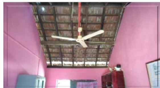
Repairs to school building and painting Perunawalar College Alayadiwambu Divisional Secretary Division Ampara District
