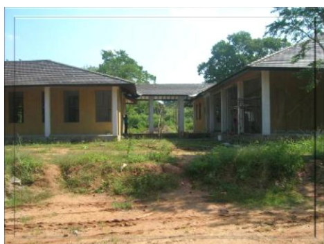
Animal Hospital being constructed
