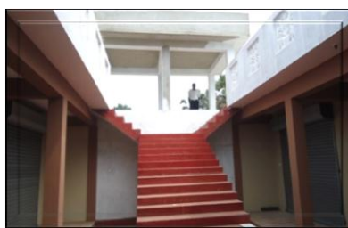
Construction of Talai Mannar Market Complex, Mannar District
