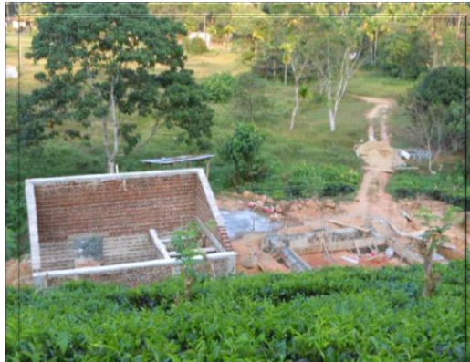
Construction of Sanitary facilities
