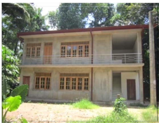
Community Hall constructed in Minuwangoda Divisional Secretary Division, Gampaha District
