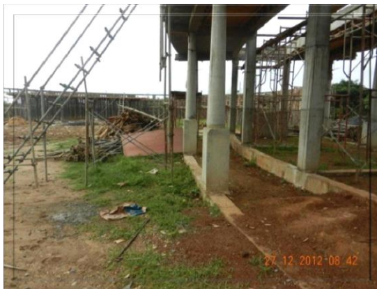
Construction of Main Entrance
