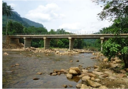
Reconstructed MalalpolaPiduruwella Bridge Yatiantota DS Division Kegalle District
