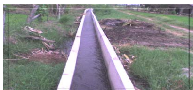
Concreted Balance section of 9C Field Canal, Hambantota Divisional Secretary Division Hambantota District
