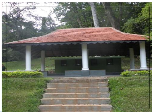
Re-Construction of summer huts
