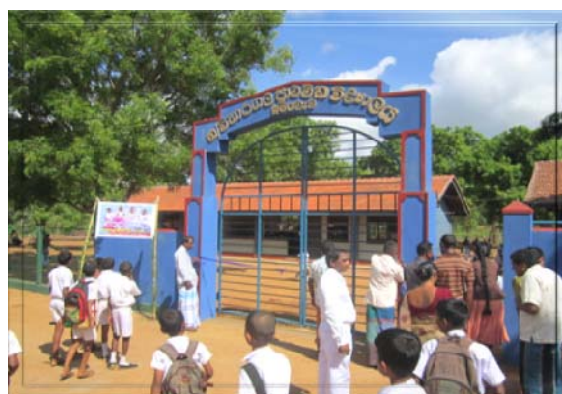
Reconstructed Fence and Gate Viharagala Primary School, Suriyawewa Divisional Secretary Division, Hambantota District
