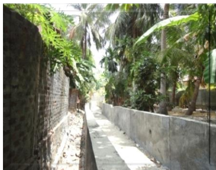
Construction of water Supply project Trincomalee District
