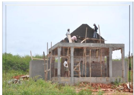
Construction of summer huts
