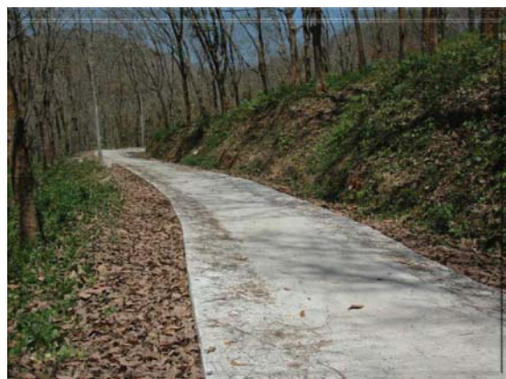
Road constructed Pananawatte at Warakapola Divisional Secretary Division Kegalle District
