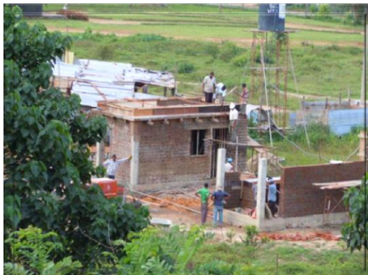
Construction of ticket counter
