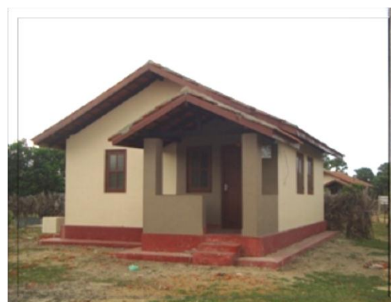
Indian Pilot Housing Scheme - Mullativu District
