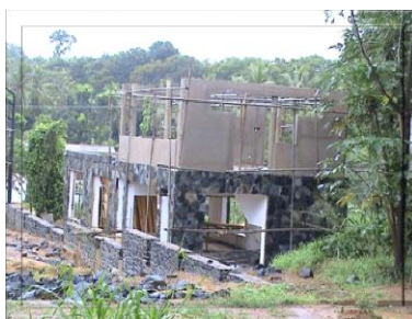
Souvenirs shop being constructed
