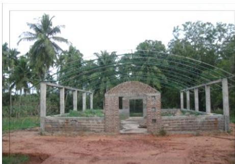
Construction of plant houses
