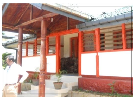
Improved Bagawantalawa Rest House
