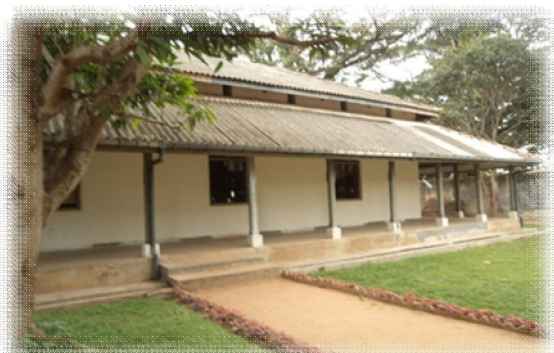
War Hero Resource Centre which is being constructed in Hedala, Hekiththa
