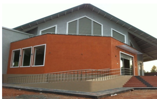
Lecture hall constructed at Makandura center.
