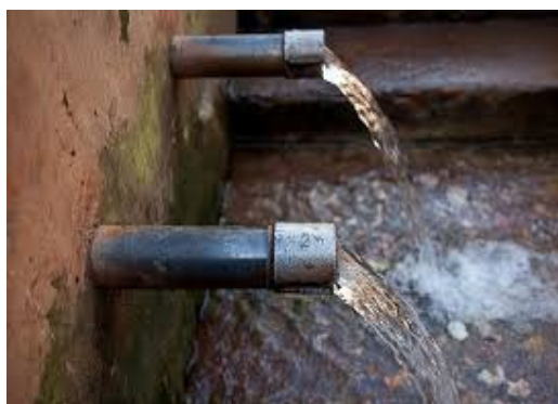
Pipe line Watering
