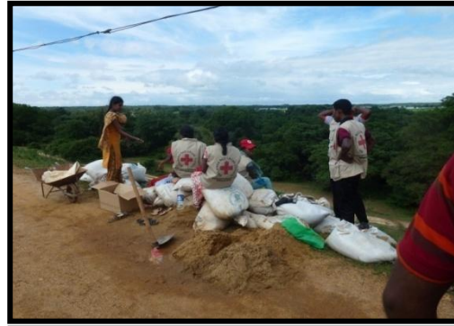
Placing the sand bags to control the ooze of water in Iranaimadu bund with the aid of SLRCS volunteers
