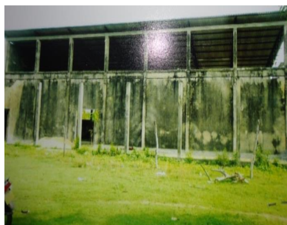
Repairing of Paddy Store at Thoppur By Dayata Kirula - 2013
