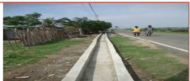
Construct 225m Drainage Channel with one Culverts Connect with Existing Cannel from Rajalikulam
