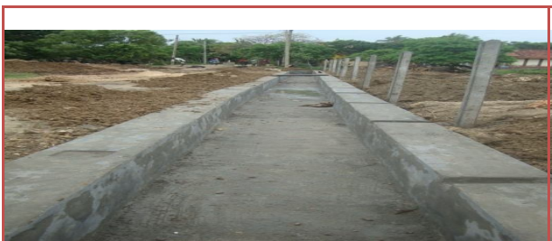
Construction Drainage System at Sakkodai
