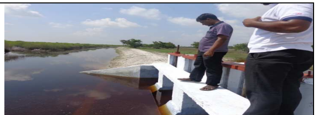
Flood Mitigation Project at Ampan
