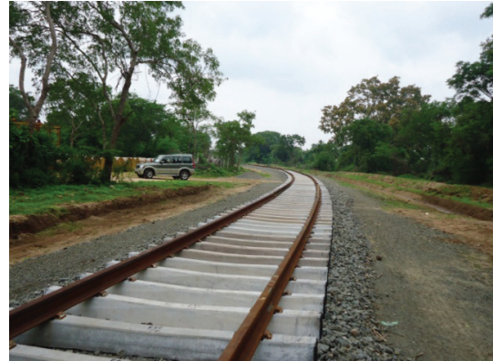
Railway line development activities under reconstruction of Northern Rail roads Programme
