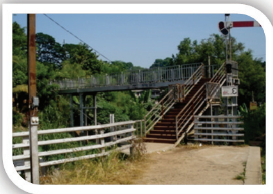
Peradeniya overhead bridge.
