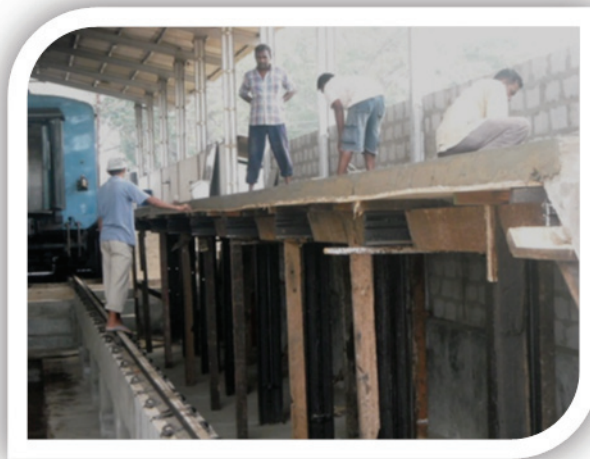
Renovations to Colombo Running Sheds are underway.
