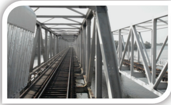
Construction of dual railway line up to Kaluthara South.
