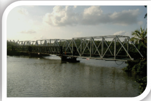
A photograph taken while the Ja-ela bridge is being rehabilitated.
