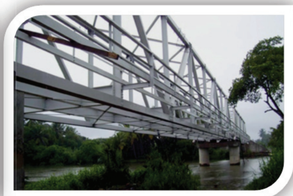
Matara Nilwala bridge.
