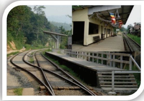
Geli- Oya Railway Station after improvement.
