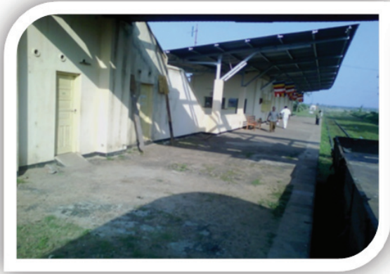
Newly Constructed Punanai Railway Station.
