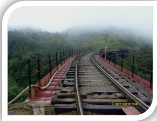
A view of the Ambewela bridge after rehabilitation.
