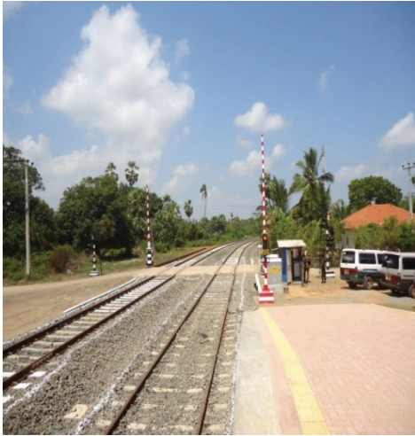
The protected gates constructed in the Northern line.
