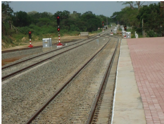
The completed Madawachchi –Madu Line
