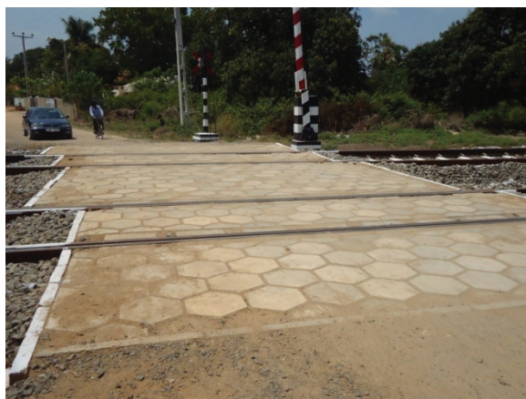
Construction of protected railway level crossings
