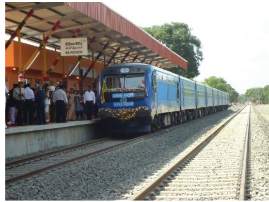
The newly constructed Kilinochchi Railway station
