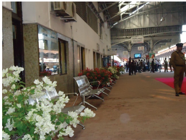
The renovated Fort Railway Station
