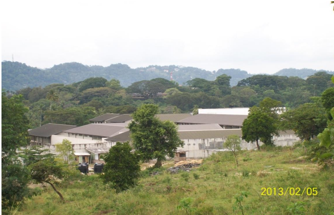
A part of new prison complex at Pallekele due to be opened in the near future
