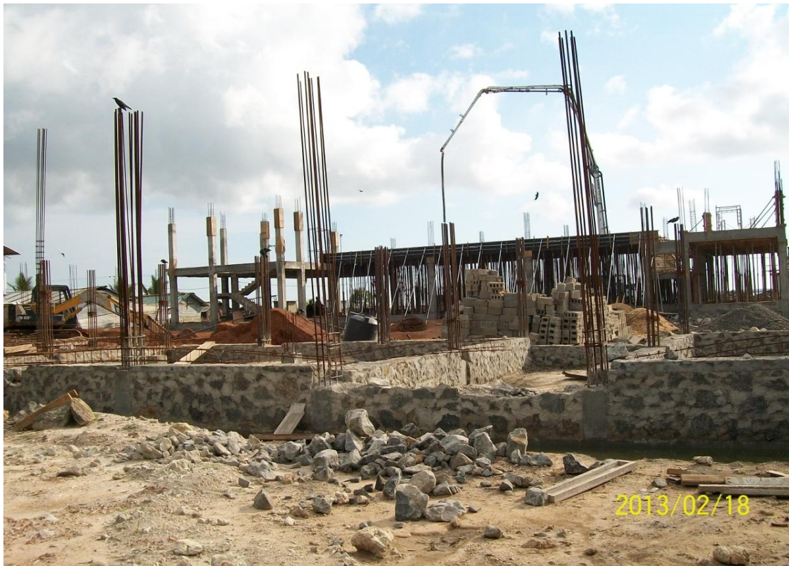
On going constructions of Jaffna Prison Complex
