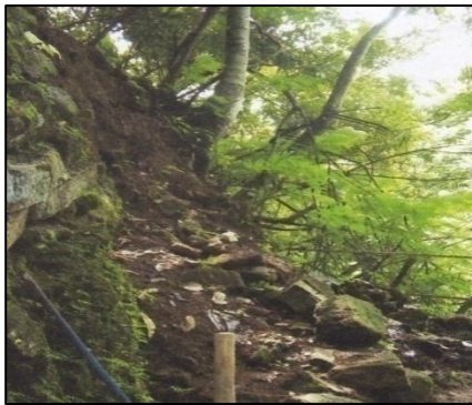
Rampart on the right before maintenance
