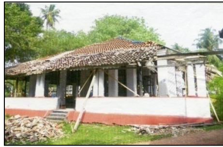
The manner of roof was conserved
