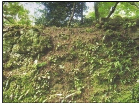
Rampart on the left before maintenance
