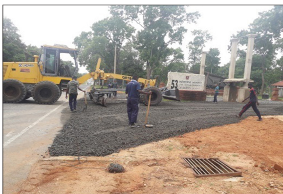
Disaster Management Assistance to public transportation at Kiran by 23 Division during the flood sits on 03 November 2017
