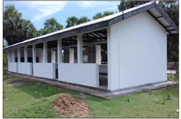
Renovation of school building at Wallawadiya Sinhala Maha Vidyalaya, Batticaloa on by 23 Division
