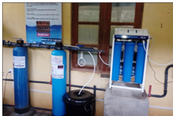
Installing Reverse Osmosis Plant at Headquarters premises of 61 Division
