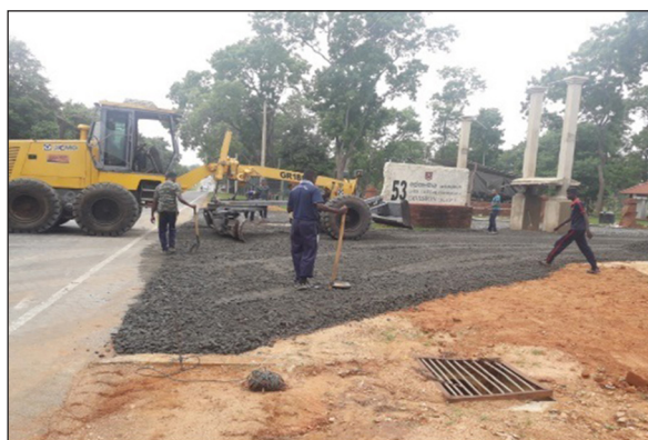
Assist to road development project at Inamaluwa
