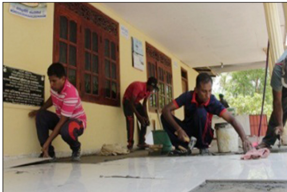
Construction of Sangawasaya of Jayanthipura Temple by 10 Battalion the Gajaba Regiment
