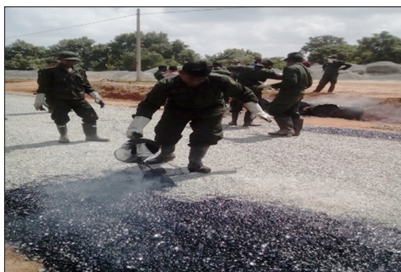
Construct road of Punani Regional Ordinance Stocks Complex (ROSC)
