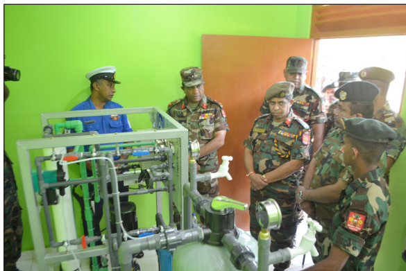
Construction of water purification systems
