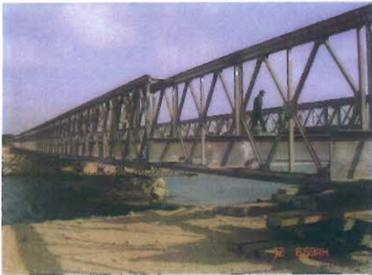
BRIDGE AT THONDAMANARU ROAD
