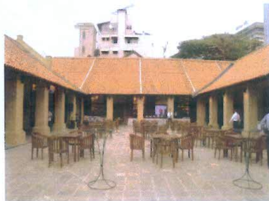
RENOVATION OF OLD DUTCH HOSPITAL COLOMBO
