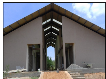
Staff utility building being constructed
