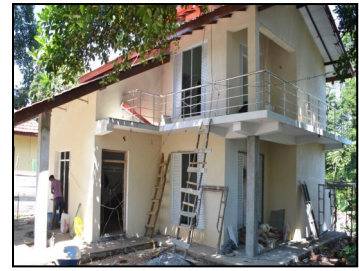
Newly constructed house
