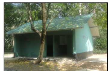
New lavatory system
