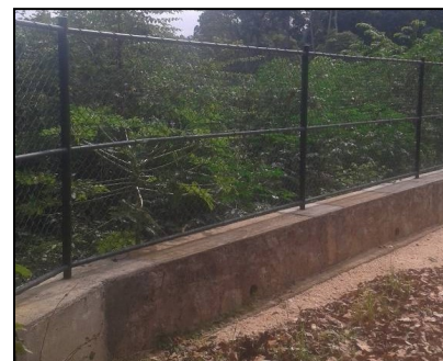
Boundary wall next to office
