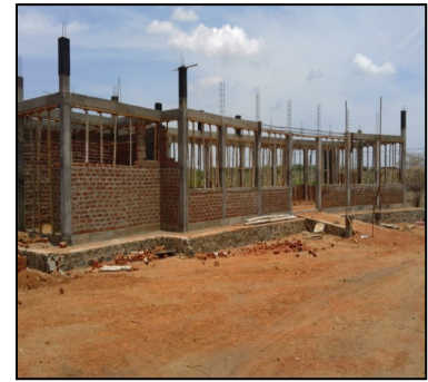
New canteen for visitors – constructions on going
