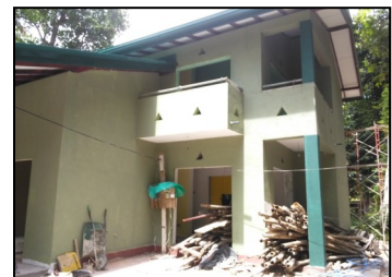
Newly constructed quarters
