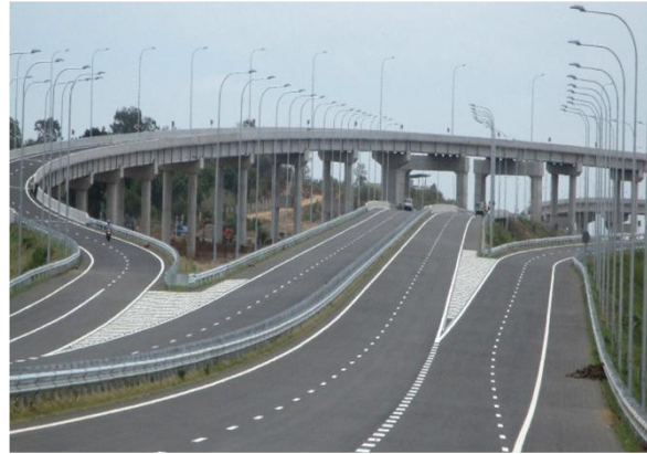
Extension of Southern Expressway Section 04
