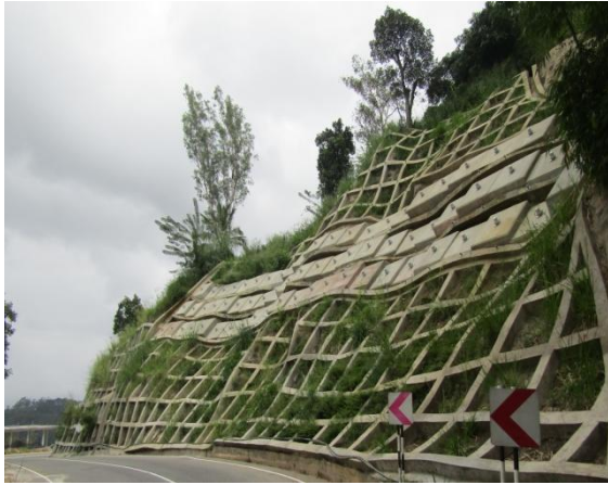
Construction of crib work and ground anchor work
