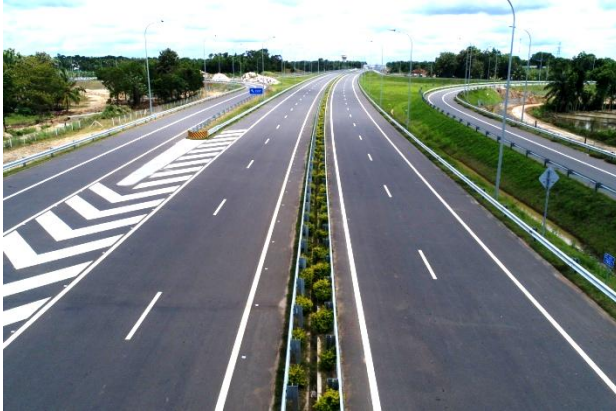
Extension of Southern Expressway Section 03
