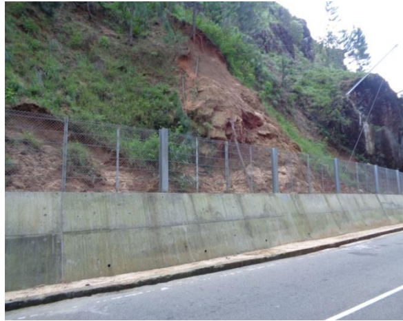
Construction of Rock Fence
