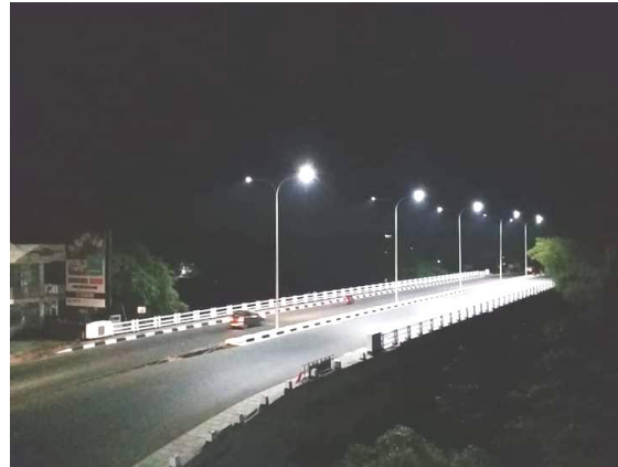
Reconstruction of 25 bridges Project – Package 01, Bridge No. 1/1 on Kaduwela – Biyagama – Road
