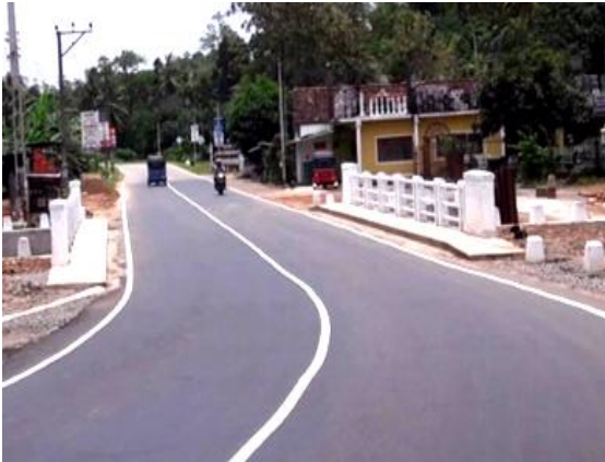
Reconstruction of 25 bridges Project – Package 01, Bridge No.14/3 on Galagedara – Horana Road
