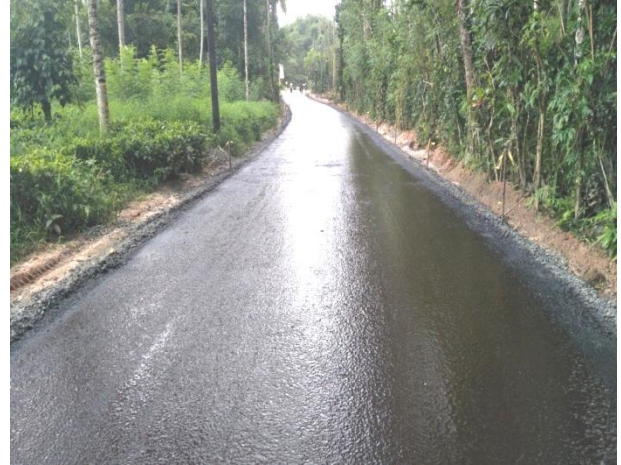
Priority Road Project – Phase II, Kannaththota – Ihalagama Road (Asphalt Paving)
