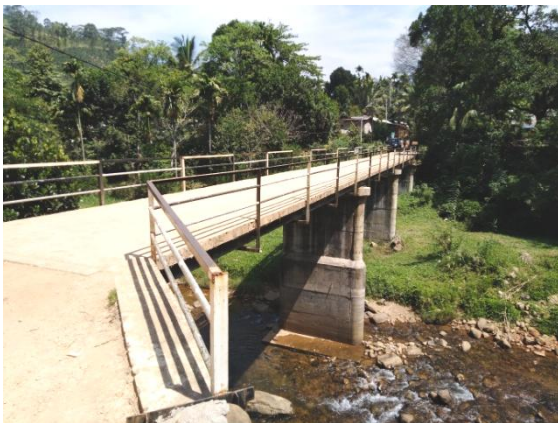
Rural Bridge Construction Project- Nawalapitiya Greenwood Bridge in Kandy
