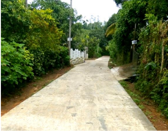
Road in Galle- Karanadeniya Kusalakanda Village
