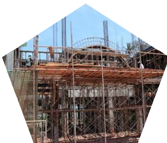
Constructions of Seeduwa building complex
