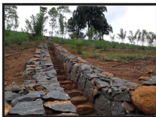
Land Preparation for 2 nd Subsidy Payment
