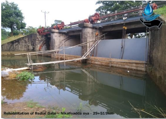
Rehabilitation of Radial Gate - Nikallyadda oya - 29+51.9km
