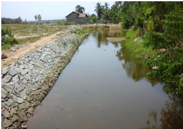
Rehabilitation of canal in Akkaraipathu unit
