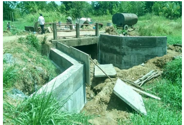
Construction of Chainage 4+892Km in Muthukandiya scheme in Moneragala
