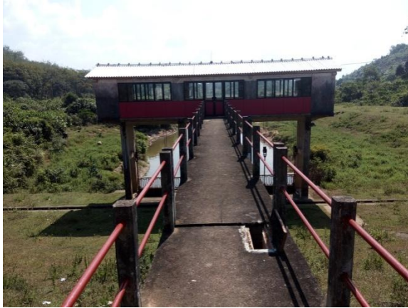
Divithura Flood House Aluminium Works
