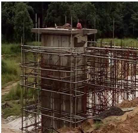
Construction of LB Sluice
