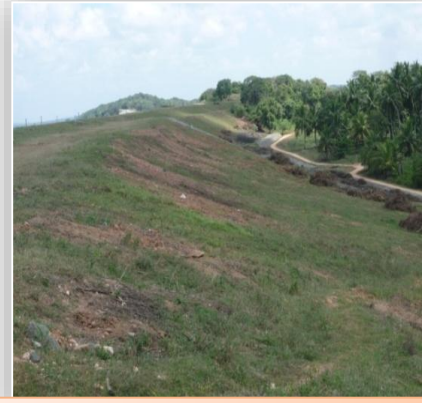
Clearing & Weeding Kaudulla Tank Bund under O & M Gravity works
