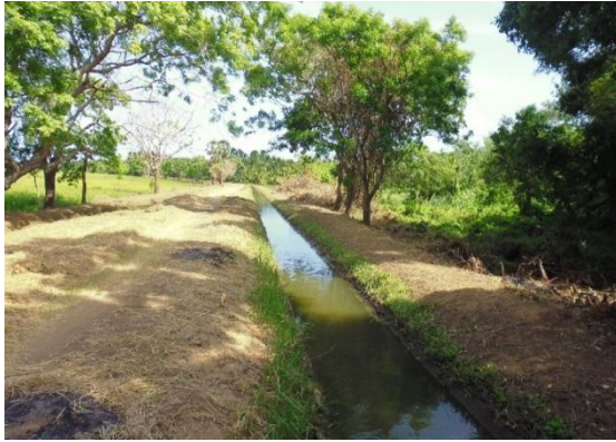
Distributory Canal maintained by Sharamadana under social security Program of Dam Safety Project - Maha Wilacchchiya Scheme
