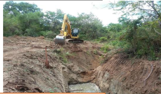
Excavated area of Debaraara feeder canal
