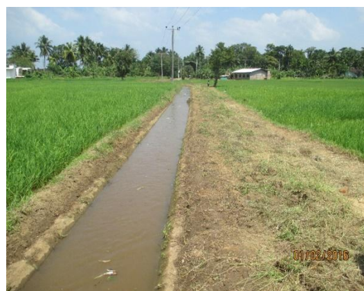
A canal with regular maintenance Minipe Scheme
