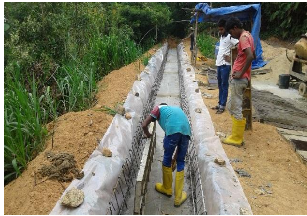
Construction of toe drain at Galkanda Kanista Vidyalaya
