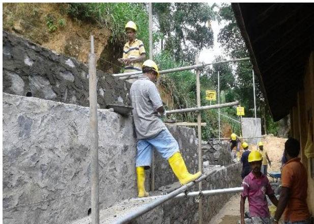
Construction of retaining wall at Galkanda Kanista Vidyalaya
