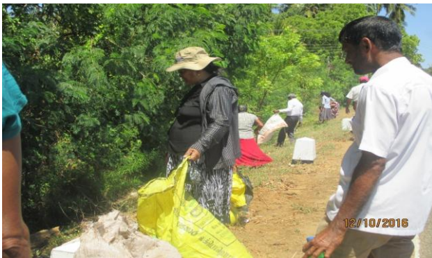
Removing garbage and waste in irrigation canal Kiridiyoia scheme
