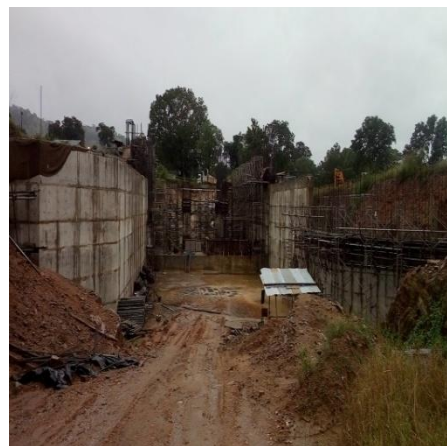
Construction of Spill
