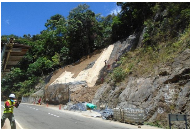
Slope stabilization and removing of falling rocks in Kandy Mahiyangana Road
