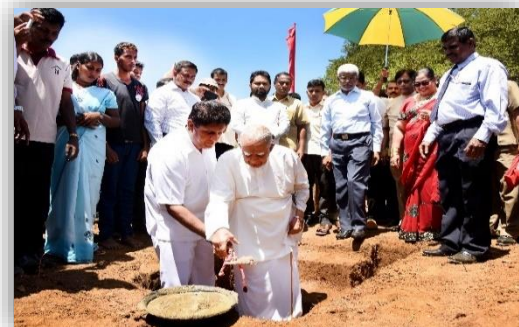
Laying foundation stone for a model village under the Northern Province housing
