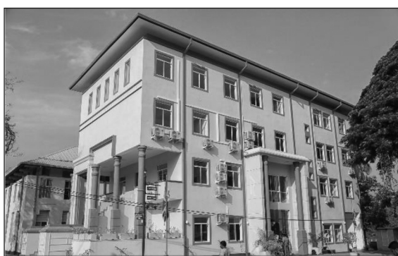
Engineering Technology Laboratory Building – Wayamba University Kuliapitiya Estimated Cost Rs. Million 282
