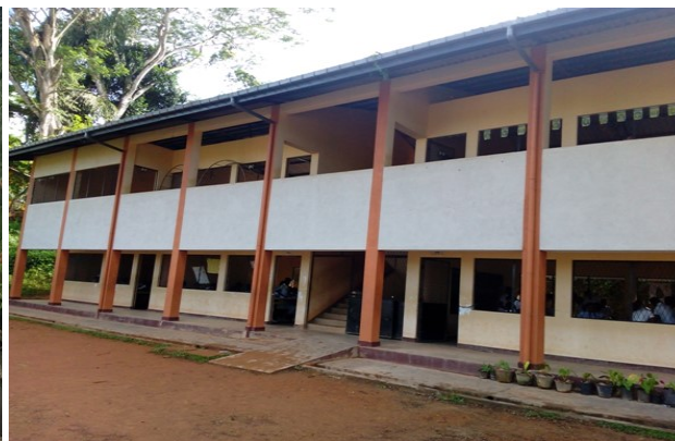
A building of Ga/Baddegama St. Anthony's College constructed under TSEP Project
