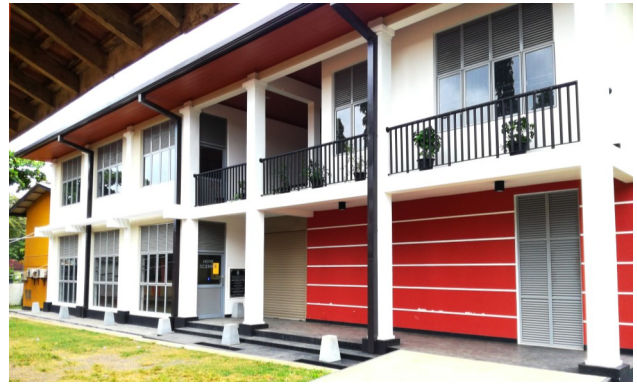
Technical Building – Kuli/ Ethungahakotuwa Central College North Western Province
