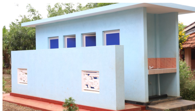
New Sanitary Facility System – Koggalla M. Vidyalaya, Hambantota – Southern Province
