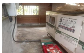
Shifting of 30 KVA Generator from SLCG 'Rohana' to Coast Guard Station
