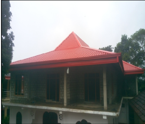
Nildandahinna Sri Abhinawaramaya – Construction of Monastery building
