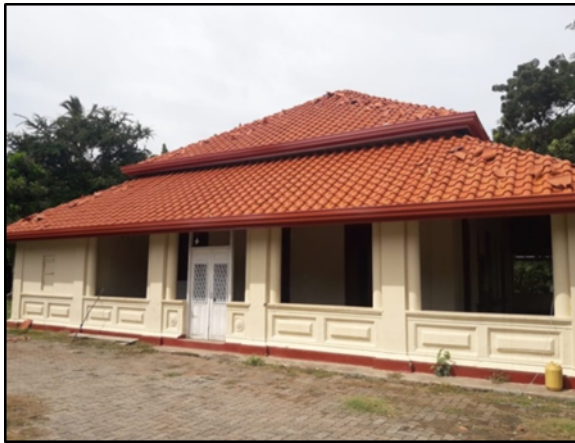
Restoration of roof of the Dhamma Shala in Rangiri Raja MahaVihara in Ambalanthota
