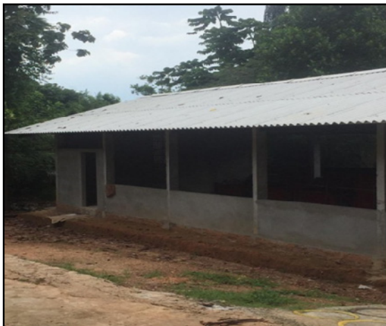
Completion of remaining works of the building of Sri Rathnapala Dhamma School in Kadawatha.
