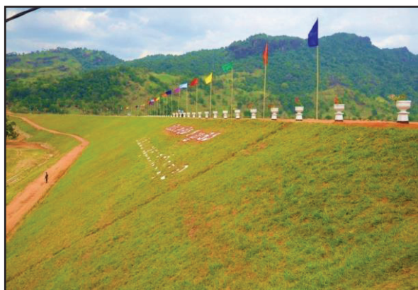
Rambukkan Oya Dam
