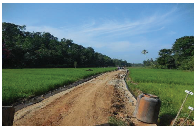
Improvement of Baddegama-Kotagoda Kanda road
