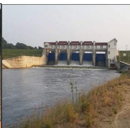
Yan Oya Spillway
