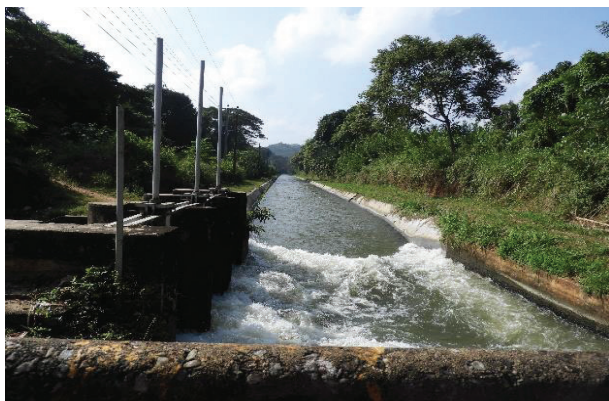
Canal lining of feeder canal from Bowatenna to dambuluoya and Kandalama
