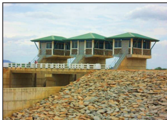
Rambukkan Oya Spillway
