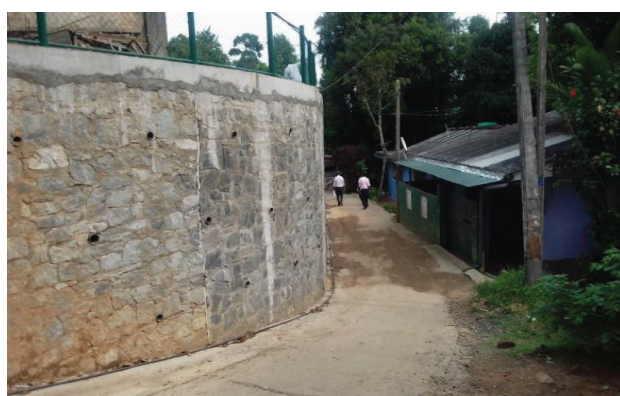
Rectification of unstable slope at Kurukuthala Muslim Vidyalaya
