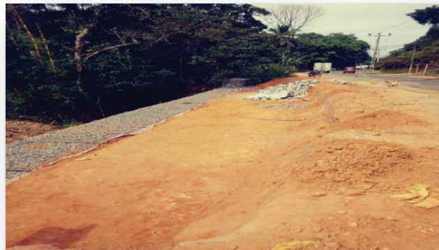
Construction of retaining wall on Thiriwanaketiya-Agalawatta road
