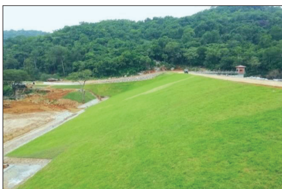
Kalugal Oya Dam
