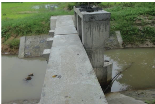
Construction of Regulator in Vahanery scheme Rugam Division
