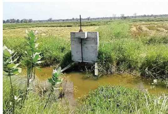
Reconstruction of Palakudi feeder tank spillway in Murunkan division
