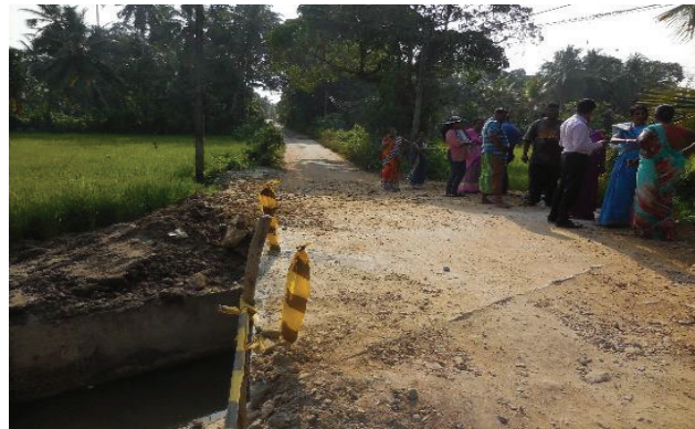
Construction of culvert on Veniwelpitiya road - Millaniya
