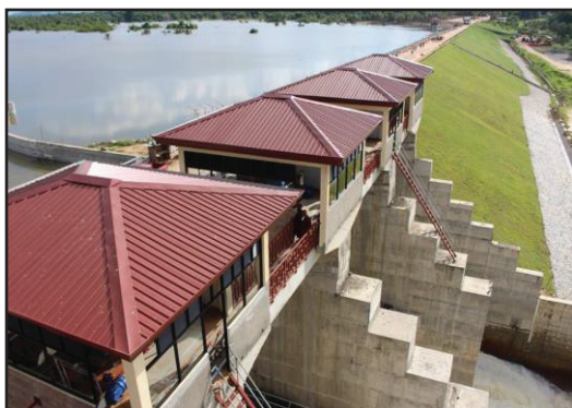
Deduru Oya Spillway
