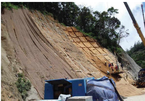
Rectification of Land Slide Along the Peradeniya Chenkaladdi Road in Haggala
