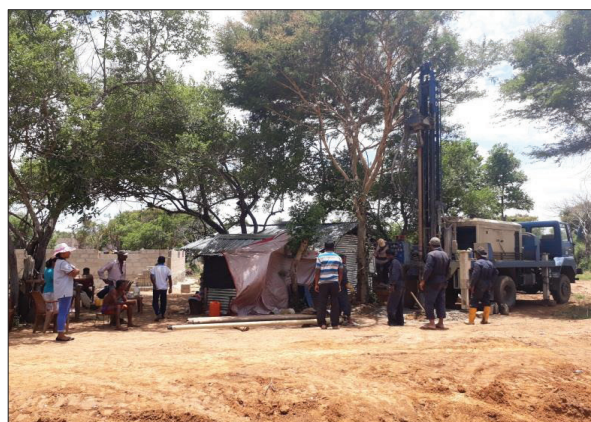
Figure 4: Construction of Tube well
