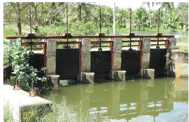
Intallation of new 79 gates for Kalawewa main canal
