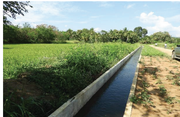
Lining of main canal- Halmullapillawea - Muthukandiya
