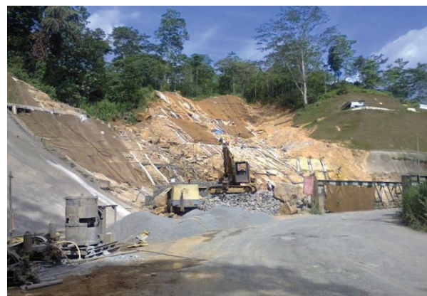
Rectification of unstable slope at bridge no.48/2 on Avissawella -Hatton Road
