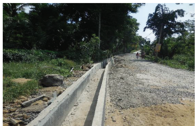
Improvement of road from Nagoda bridge to Sunandaramaya temple
