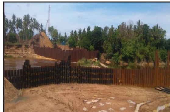
Sheet Pile Installation
