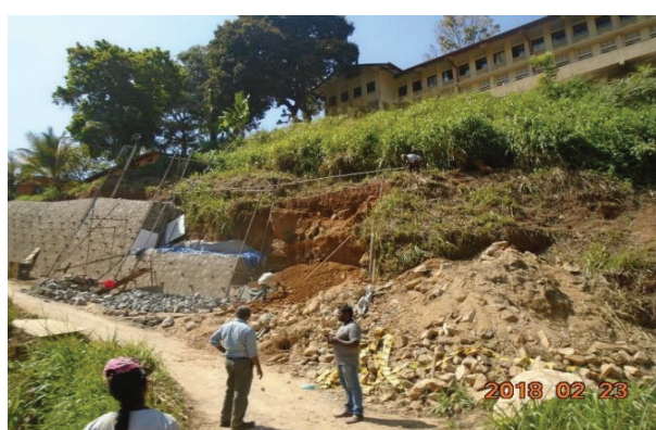
Rectification of unstable slope at Rambuke Ela Muslim Vidyalaya
