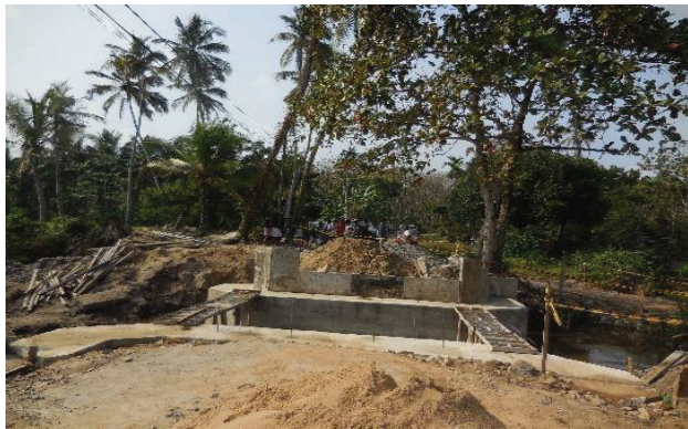
Construction of small bridge and retaining wall on Dombagoda Seelarathana road – Millaniya
