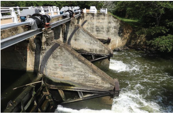
installation of 3 radial gates and geared gate operating mechanism to Ilukkwewa Anicut
