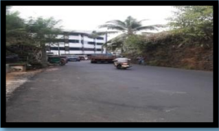
Carpetting the remaining part of Kajugaswatta road (Road Carpeting)
