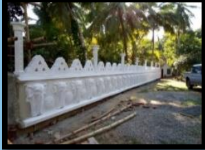
Construction of a wall around Sri Sudharmarama Rajamaha Viharaya in Thoragala,Hingura
