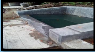
Construction of the bathing well in haththella division
