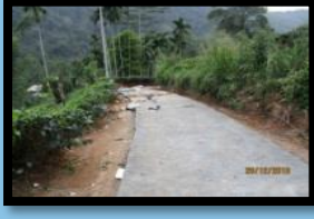
Construction of Galpoththa Henyaya road(Samurddhi)
