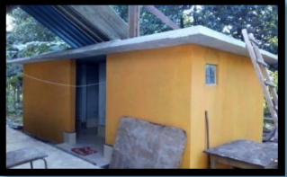
The monastery bein constructed at Sri Isipathanaramaya in Bulathwelkanda
