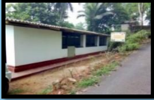
Development of the Community Hall in Millawitiya
