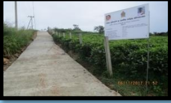
Renovation of Pitawala road
