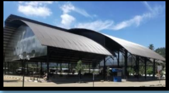
Construction of the weekly fair in Nivithigala(SRIDP)
