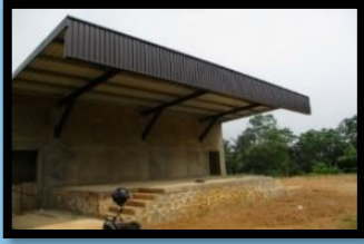
Construction of the pavilion at the Wanniarachchigama Plaground in Pelmadulla
