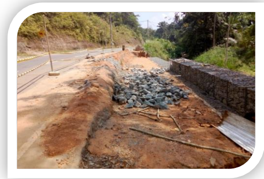
Construction of Gabian at Thiriwanaketiya. –DS Nivithigala
