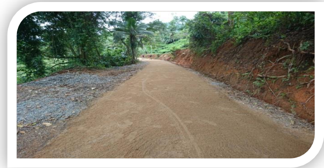
Renovating kadawatha road via Ambagahakandap Ilukpotha, Pelawatta - Kalawana DS Division
