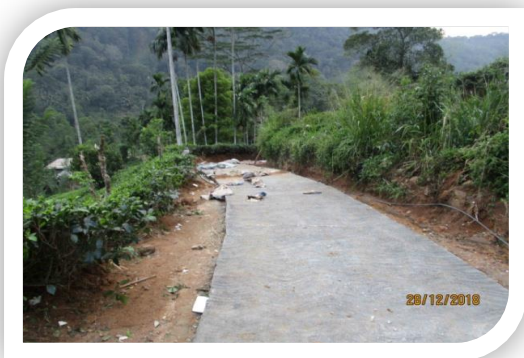
Construction of Galpoththa – Henyaya Road
