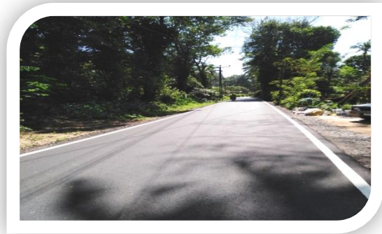
Construction of Kotamulla-Amuwela Road DS-Elapatha
