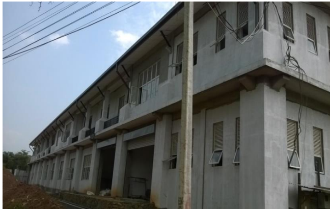
Construction of new District Secretariat Complex –Basic phase
