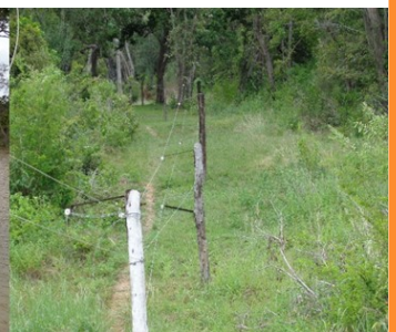
Constructing Electricity Fence
