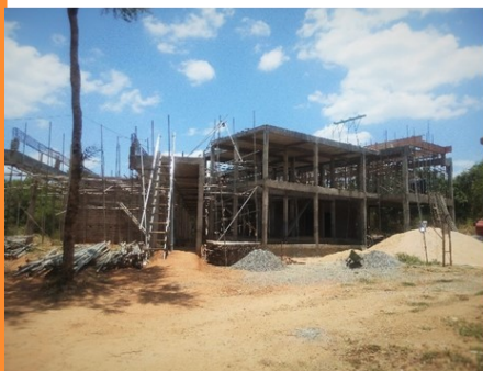
Resident Project Manager's Office
