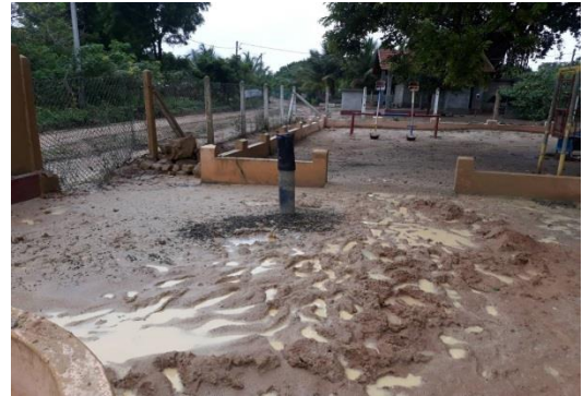
Recontionof Well to Gnaoli pre School at PTK East
