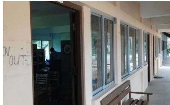
Reconstruction of Building to Barathimakaviththiyalayam Valluvarpuram
