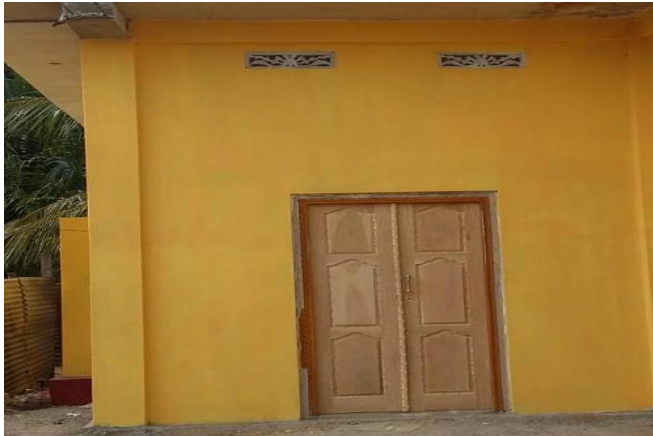
CONSTRUCTION OF NEW BULDING AT YOGAMPIKAI SAMETHA YOGAPURANATHAR ALAYAM, ANICHCHIYANKULAM
