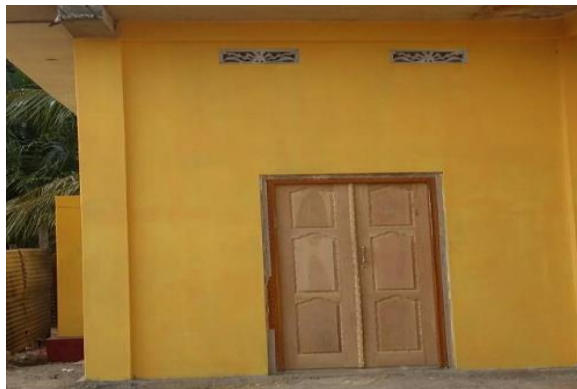
CONSTRUCTION OF NEW BUILDING AT YOGAMPIKAI SAMETHA YOGAPURANATHAR ALAYAM, ANICHCHIYANKULAM
