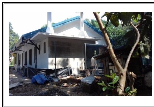
2 nd stage of constructions in Day care center
