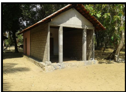
Renovation of Kodukkulachchi Iyanar
