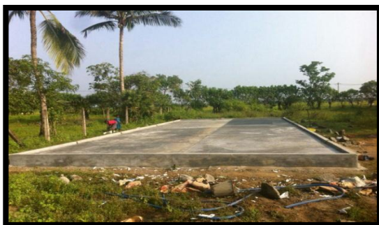
Construction of Paddy Dry stage for
