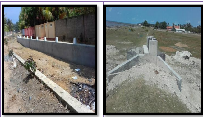
Disaster Mitigation Projects
