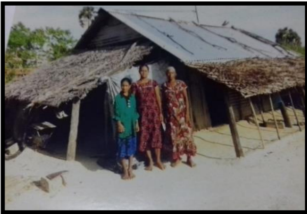
Before the Construction – Kopay
