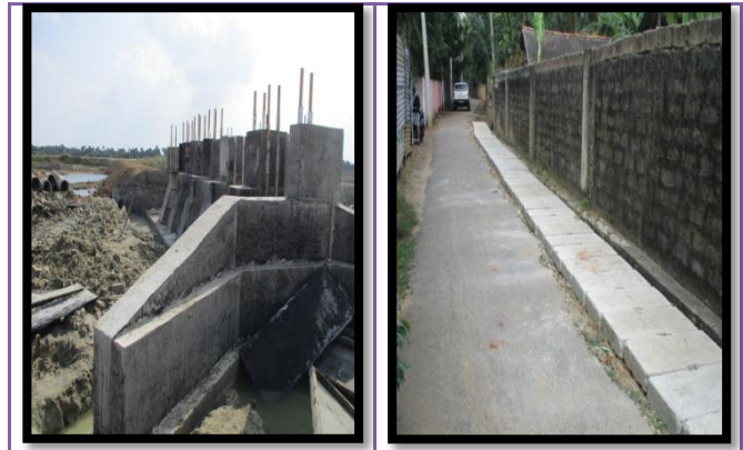
Disaster Mitigation Projects
