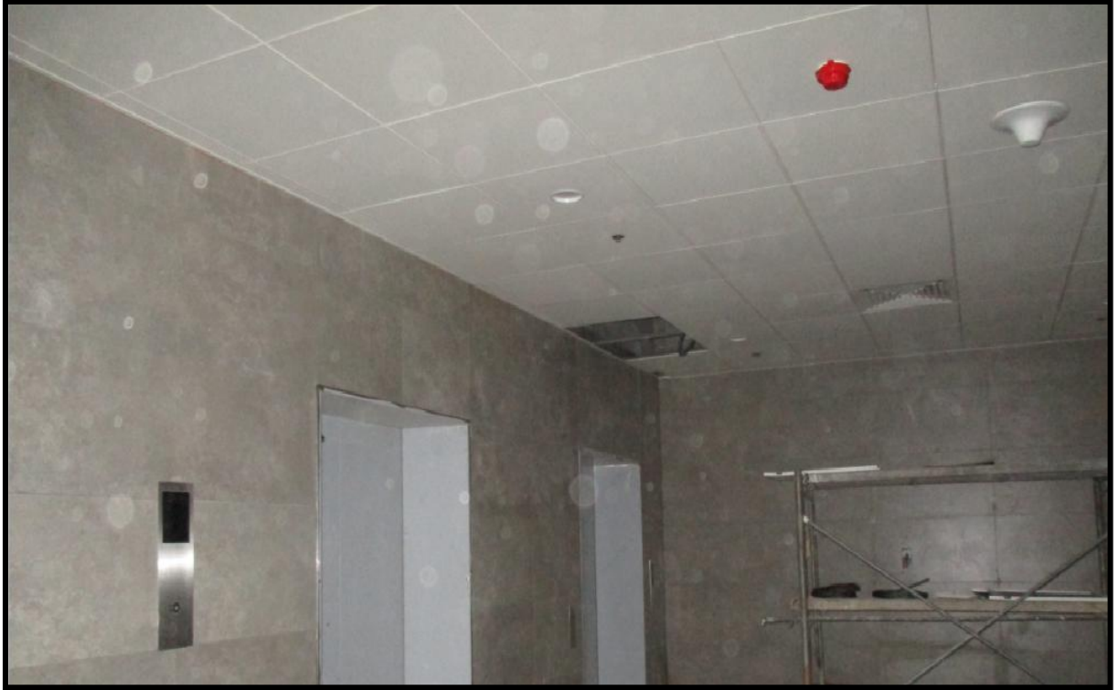
18 th Floor Lift Lobby
