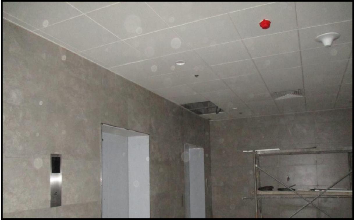
18 th Floor Lift Lobby
