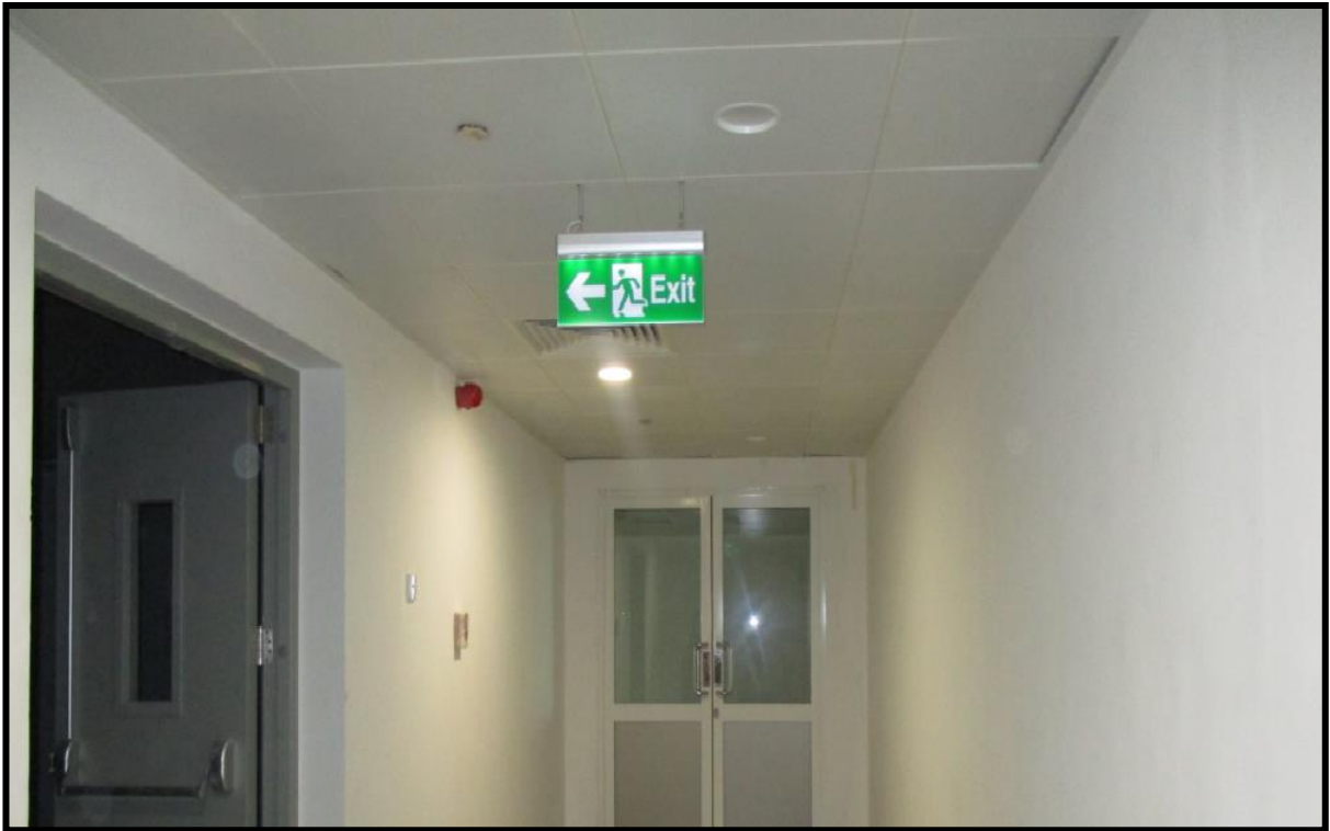
18M Floor Corridor
