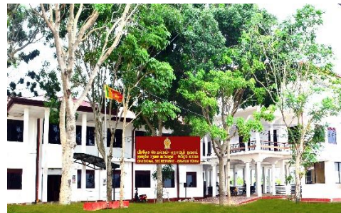
Construction of New office building at the cost of 42.8m for DS office, Eravurtown, was opened by Hon Prime Minister Ranil Wickremesinghe
