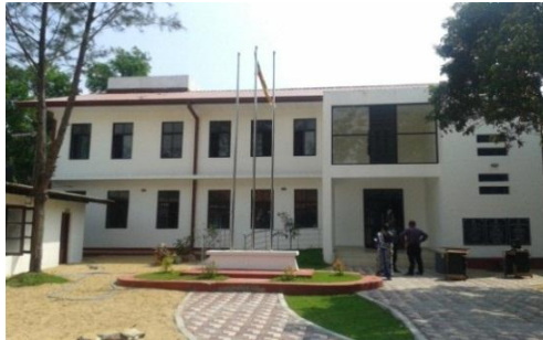
Contr. of New office building at the cost of 27.8m for DS office, manmunaipattu
