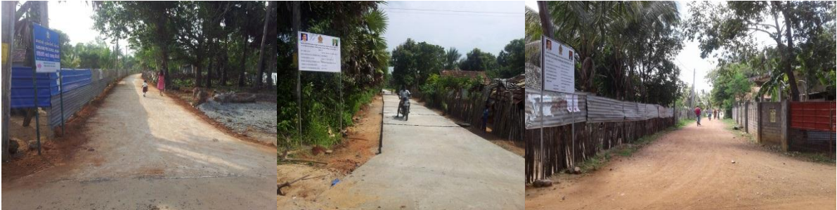
Roads & Culvert renovations- Koralaipattu South Divisional Secretariat Division
