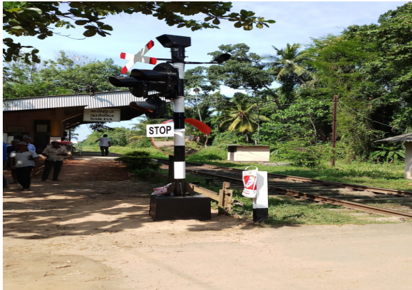
Installed signalling and alarm system near Nileeya railway station
