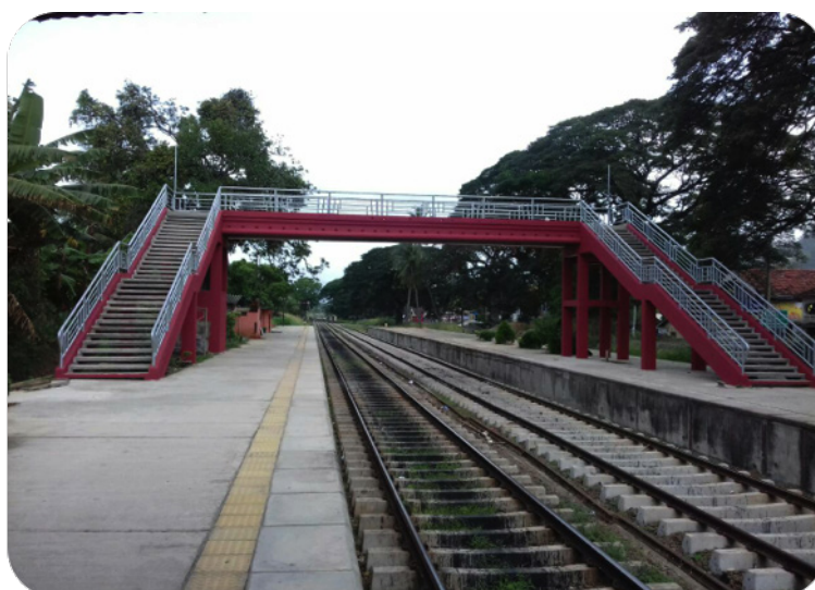
Newly constructed Platform & overhead bridge at Wellawa
