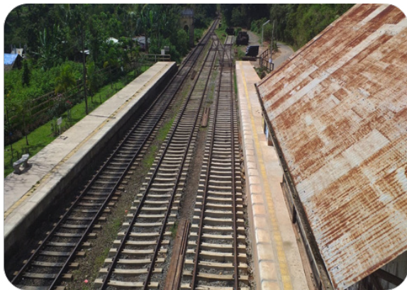
Newly constructed loop line & plat form at Ella Railway Station
