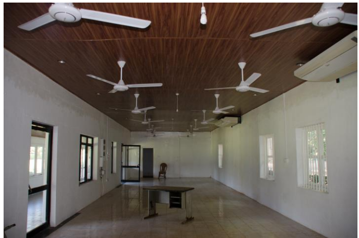
Renovated roof of the Garden cafeteria
