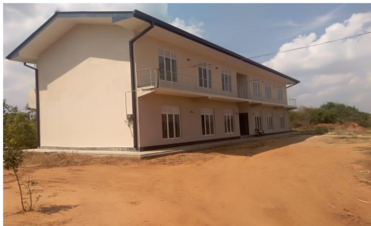
Newly constructed Housing complex with 04 quarters
