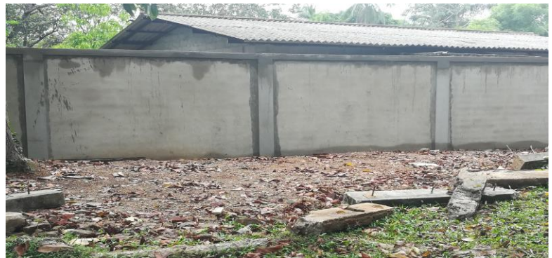
Part of the rehabilitated protective wall
