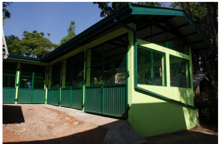
Completed building to store the garden's machineries
