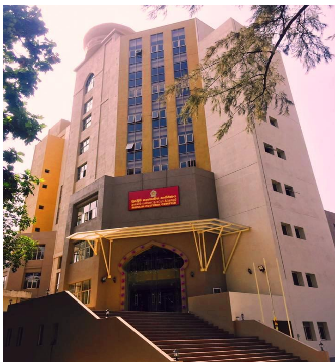
View of the Muslim Cultural Complex Building after the Construction works
