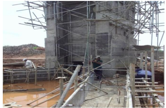
Fabricating and installing 02 sluice gates for Handapanagala Oya project.
