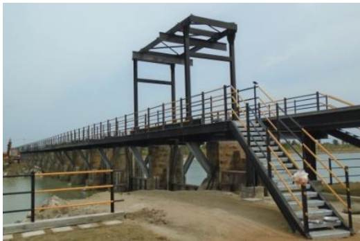
Fabricating and installing 18 sluice gates for Thondaman Aru project
