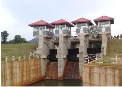
Fabricating and installing 03 radial gates for Morana Project
