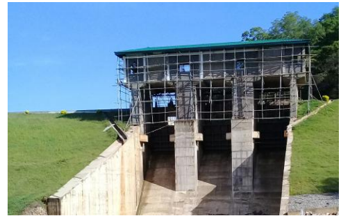
Fabricating and installing 03 radial gates for Alikota Aru – Wellawaya Project
