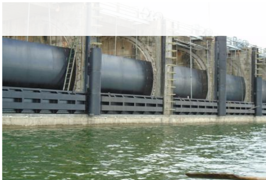
Fabricating and installing 15 radial gates and hoisting system for Rajanganaya project
