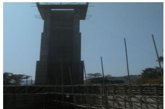
Fabrication and Installing 02 radial gates of Uva Kuda Oya project,.
