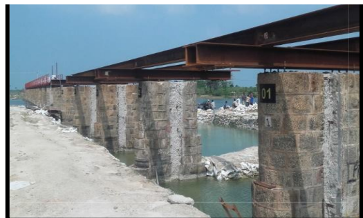
Fabricating and installing 18 Nos gates for Thondaman Aru Project.
