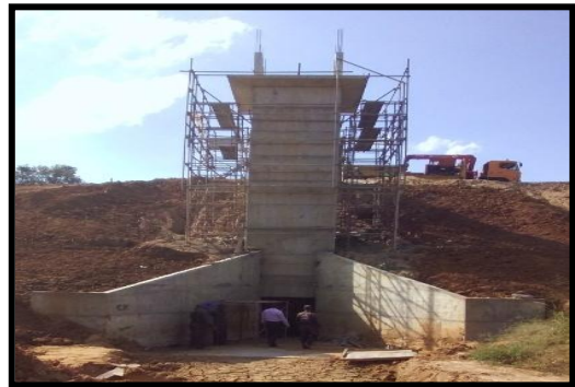
Fabricating and installing 02Nos radial gates and 01 cast iron gate for Kudaoya project, Uva
