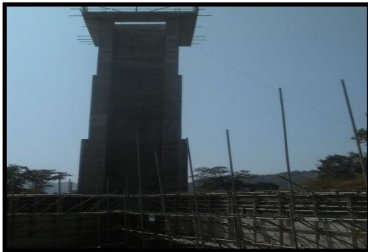
Fabricating and installing 03 Nos radial gates for Morana
