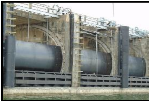
Fabricating and installing 15Nos radial gates for Rajanganaya project
