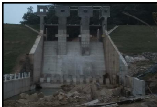
Fabricating and installing 03Nos radial gates for Alikota Aru – Wellawava Project
