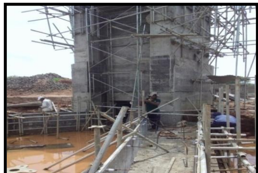
Fabricating and installing 02Nos sluice gates for Handapanagala Oya project.
