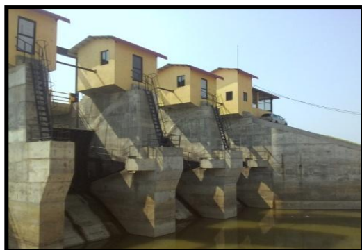
Per Aru - Fabrication & Installation of 03 Nos Radial Gate
