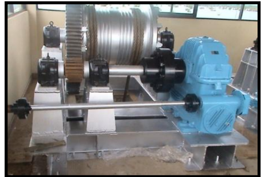
Fabricating & installing a hoising system 8 Nos Radial gates for Deduru Oya Project (As per the first plan)
