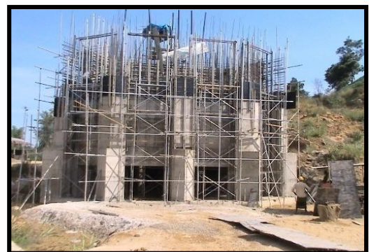
Alikota Aru Project - Fabrication & Installation of 04 Nos sluice Gates, 04 emergency Gates and 03 Nos Radial Gate at Wellawaya.
