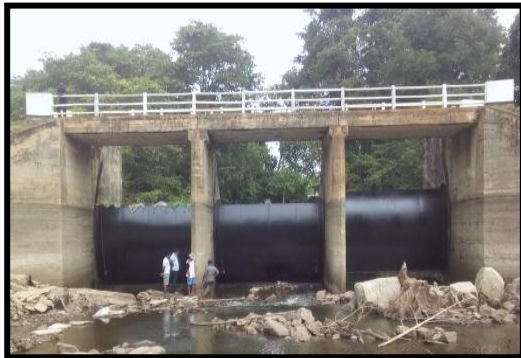
Ilukamuna Project- fabricating & installing 03 radial gates with hoising system
