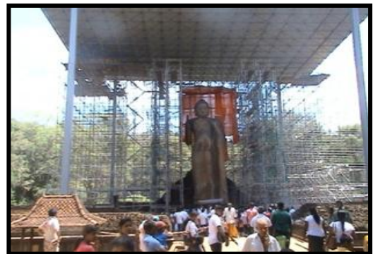
Construction of protective roof for Maligawila Buddha statue
